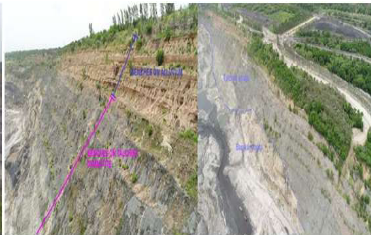
Fig. 2: South side highwall benches in the mine
