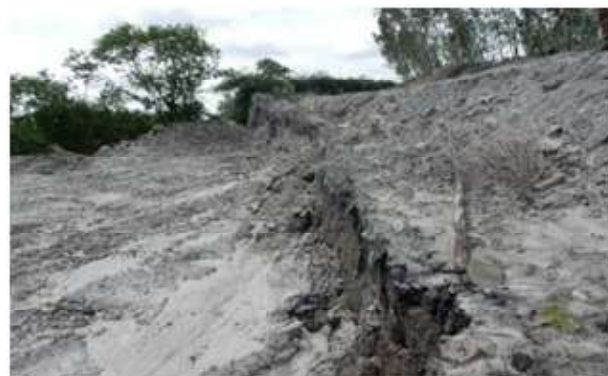
Fig. 4: Tensile cracks and vertical subsidence at surface level of highwall slope
