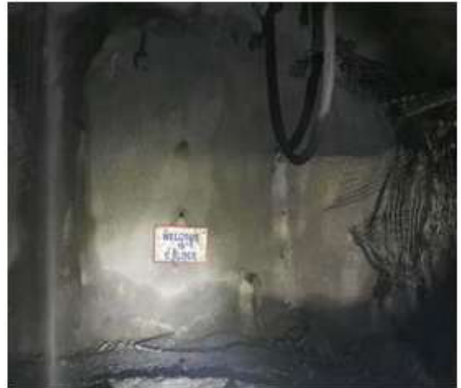
Fig. 10: A barricade constructed for paste fill plug formation (9 m height).
