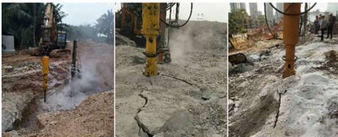
Figure 6 : Shows field use of the splitting unit
